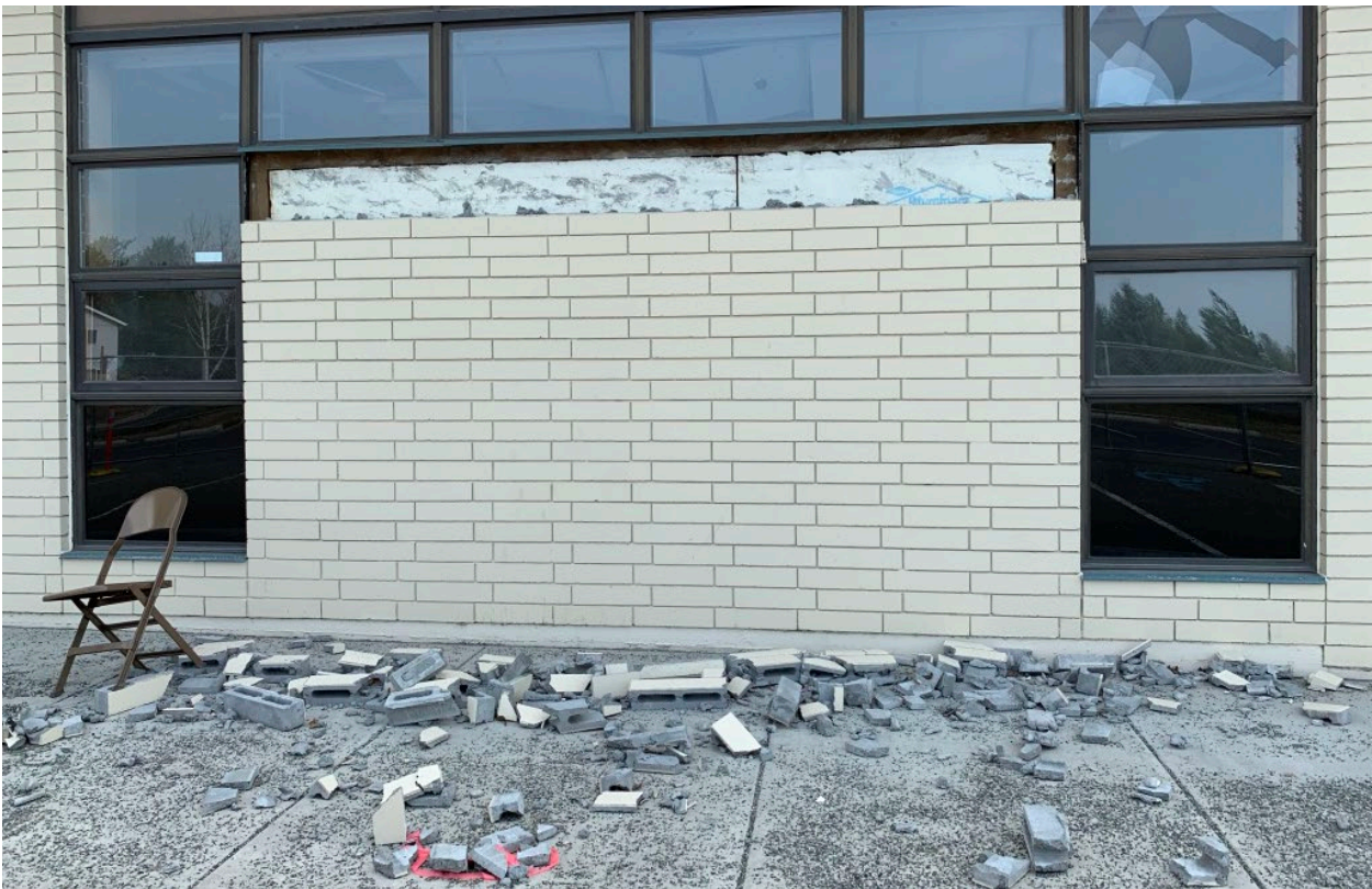
2018 Anchorage Earthquake damage to Anchorage School District, Alaska (from the Earthquake Engineering Research Institute).
